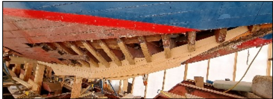
Work in progress on keel
